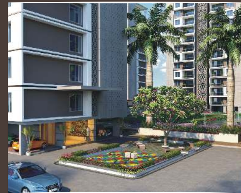
SNAKES & LADDERS GARDEN; Every structure is made with care and precision
